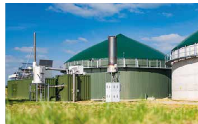
District heating generation
