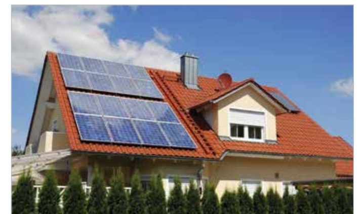
Solar heating systems (collectors)
